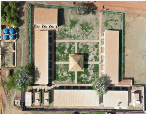
Women's accommodation cluster, UNISFA
